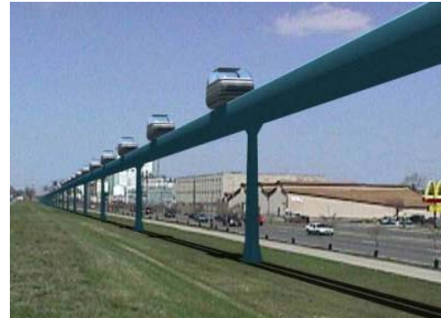
Figure A-20 - PRT Guideway and Column
