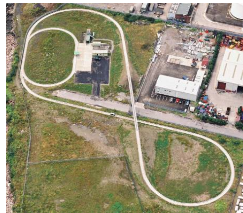
Figure 11 - ULTra Test Track Image Courtesy of ATS
